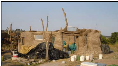
The home which is being built from recycled materials. The logs have been cut by area beavers and are being used here.
